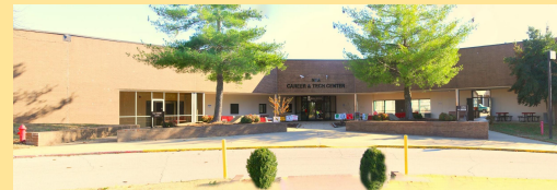
Northeast Arkansas Career & Technical Center
